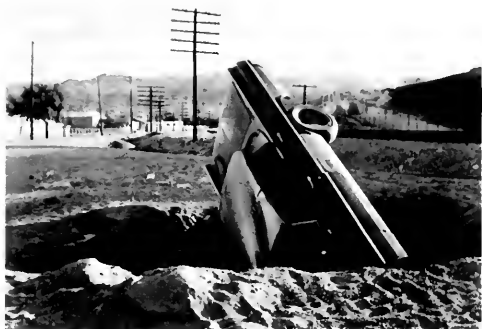
Photo 9. An 8-foot-deep crater created when a gas main blew up on Pine Avenue just south of San Fernando Road, Newhall. Main blew during first strong motion from the earthquake but fortunately did not catch fire. The car slipped into the crater as the walls began to slide back into the center. Photo courtesy of the NEWHALL SIGNAL.
